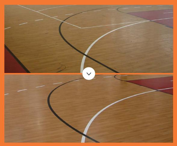
Worn sports floors can also be refreshed by applying new lines and a transparent on-top coating, without changing their original designs.
