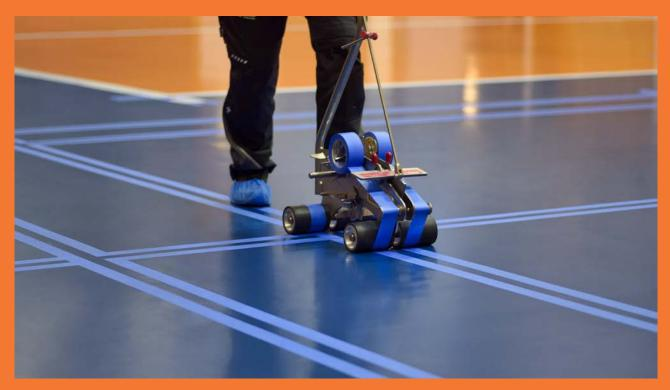
Lines are refurbished during the renovation and then permanently protected from fading and scuffing with a transparent on top coating.
