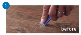
Preparation with Scraper Remove rough edges with plastic scraper.
