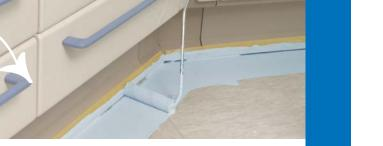
2) Lacquering the edge areas | After an intensive strip-cleaning the floor can be coated, either with a coloured or a transparent lac-quer. according to your wishes.
